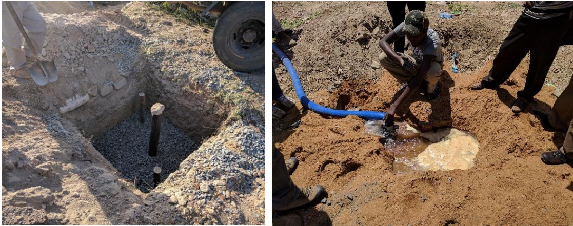
Figure 6: The Sponge Infiltration Pit demo was installed in gully along a dirt road to test the infiltration capacity of a small scale in-situ infiltration site.
